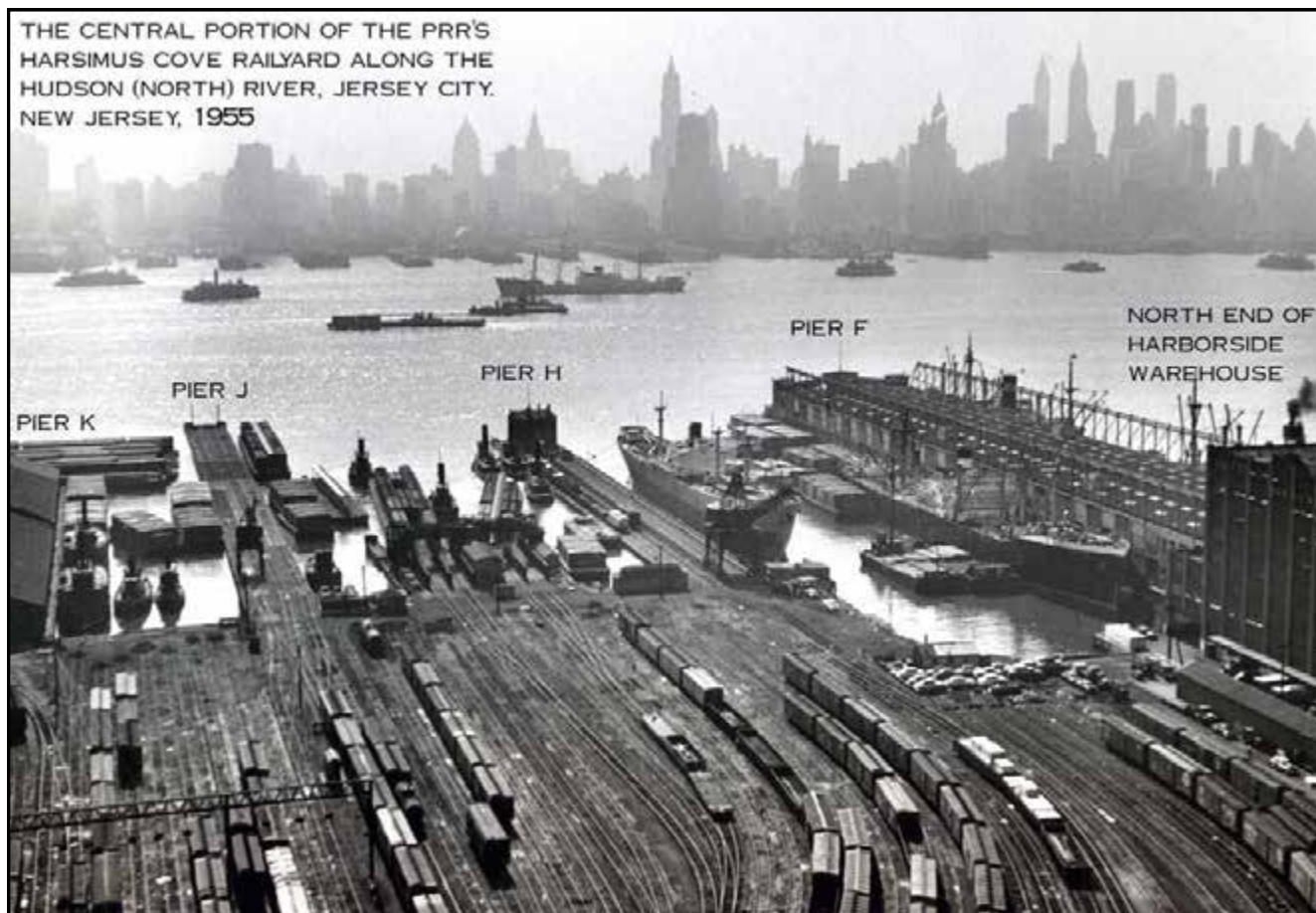
Pennsylvania Railroad Harsimus Cove Yard, Jersey City, NJ. In this 1955 image, the Yard is virtually unchanged from its wartime appearance: the central portion of the Harsimus Cove freight yard spreads out along the North River, from Pier F (from right to left) to Pier K. The right-of-way leading to Pier J was the location of the pre-positioned passenger consist used to haul German prisoners of war westbound on the afternoon of 12 April 1945. Adapted from an image in the Pennsylvania State Archives.
