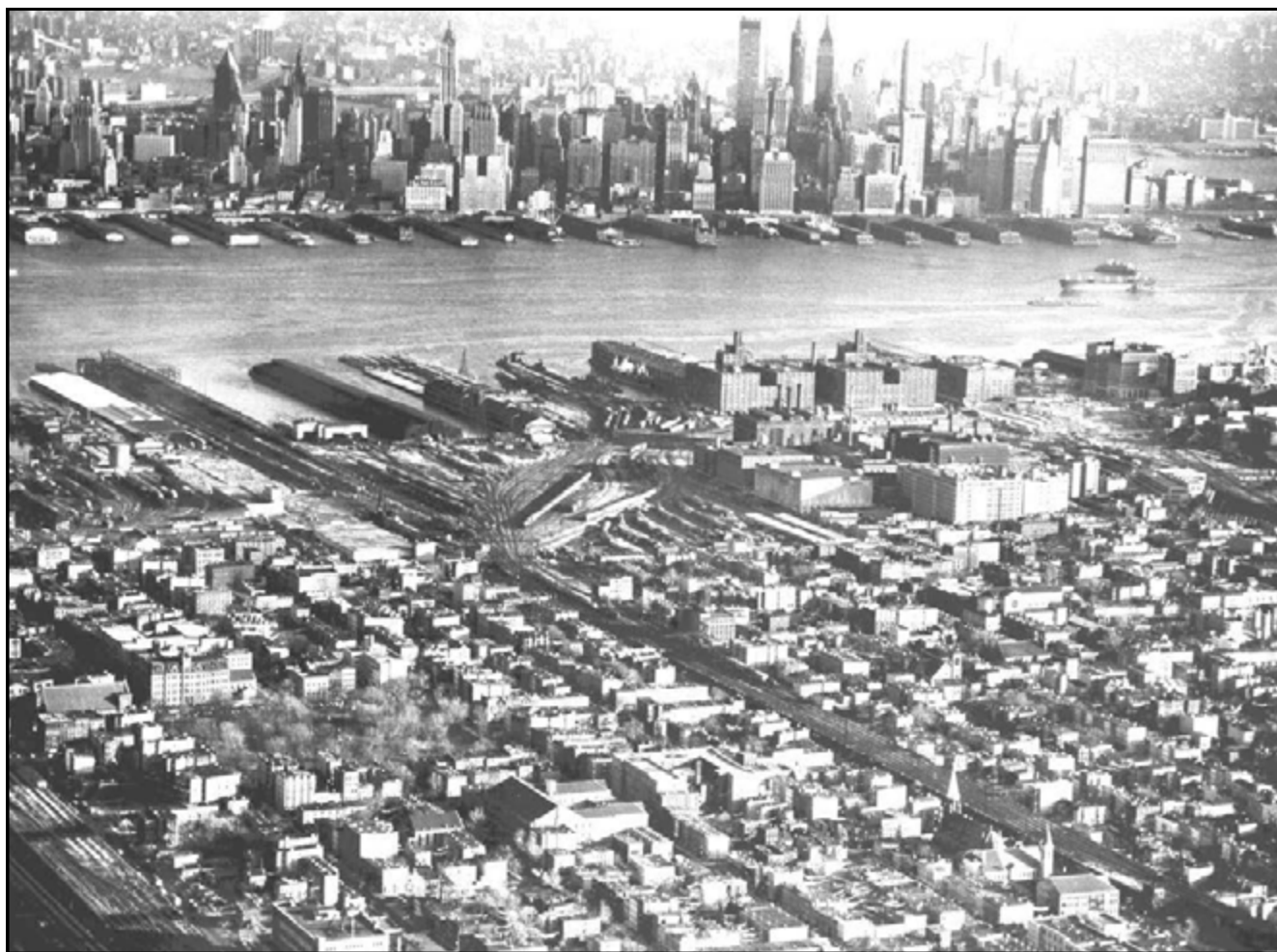
Harsimus Stem Embankment and the PRR Freight Yard, Jersey City. Diagonally bisecting this image, the Harsimus Stem Embankment, an elevated stone conduit 100 feet wide and six blocks long, facilitated the east - west linkage through downtown Jersey City between the Meadows classification yard in South Kearny with the Harsimus Cove Yard on the North River. Also in view along the River is the PRR’s massive Harborside Terminal and, across, the skyline of Lower Manhattan. Jersey City Public Library.
