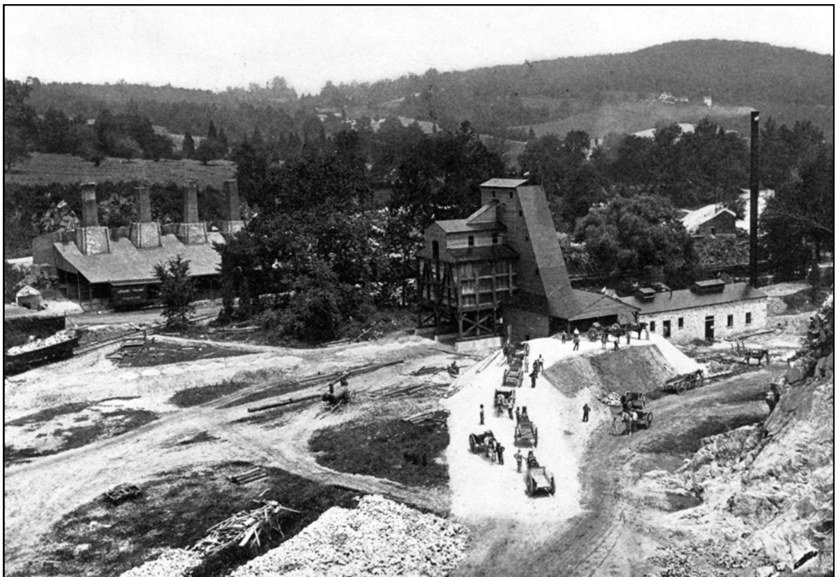
Above, the 1000 ton per day stone crusher of the Cedar Hollow Lime Company, circa 1900. A line of horse-drawn carts waits to be loaded. The quarry face is in the upper left of the photograph. Below, another view of the stone crusher, with the east kilns at upper left. Both photos courtesy of the Warner Company, 1900.
