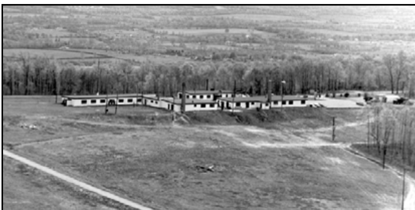
A 1963 oblique view looks southwest upon the buildings at the IFC site, which include (from R to L): the motor pool, guard shack, Administration Building, Mess Hall, NCO barracks and BOQ (Bachelor Officer Quarters), and the elongated enlisted barracks for the radar platoon. Courtesy of Chris Milewski.
