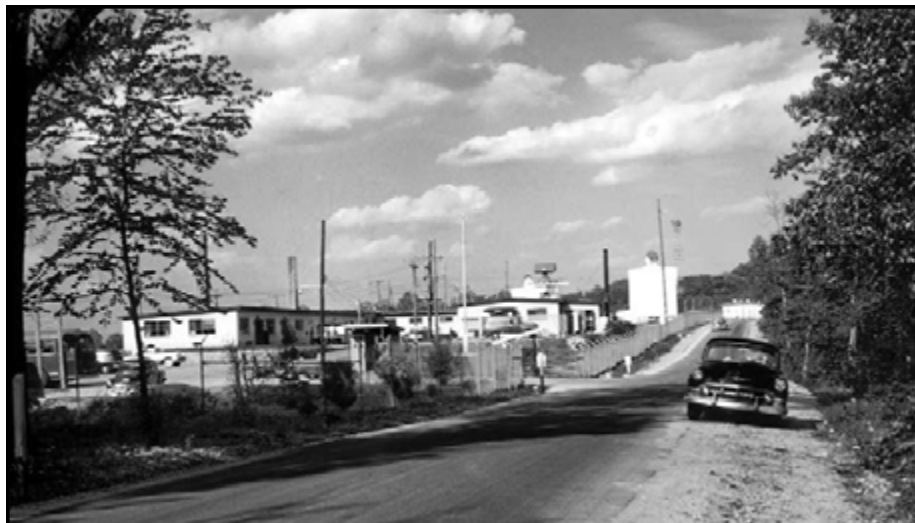
Looking east toward Valley Forge State Park along the Horse Shoe Trail in June 1959. This once unpaved logging road was improved after the Army arrived in 1955, and finally paved in 1958. Courtesy of Tredyffrin Easttown Historical Society.
