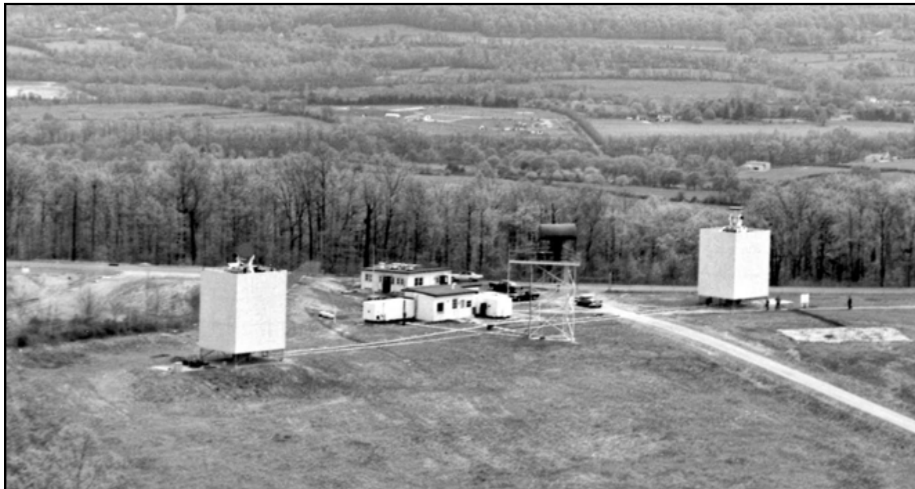
A 1963 low-altitude oblique view from the back of the IFC looks south at the two white tracking radar towers, the acquisition radar in the middle, and the small support buildings and portable trailers. What is remarkable about this image is the clear visual connection to the launch site 1.36 miles distant in the Valley below. The road running diagonally on the right connected the Horse Shoe Trail with the Army's waste treatment plant. Courtesy of Chris Milewski.
