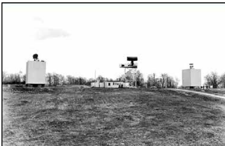
Looking southeast from the IFC area, the three radar towers are (from L to R): the target-tracking radar (TTR) to lock onto one prioritized target; the acquisition radar (LOPAR) to prioritize many incoming targets; and the missile-tracking radar (MTR) which guided the intercepting missile precisely to its target. Courtesy of Chris Milewski.
