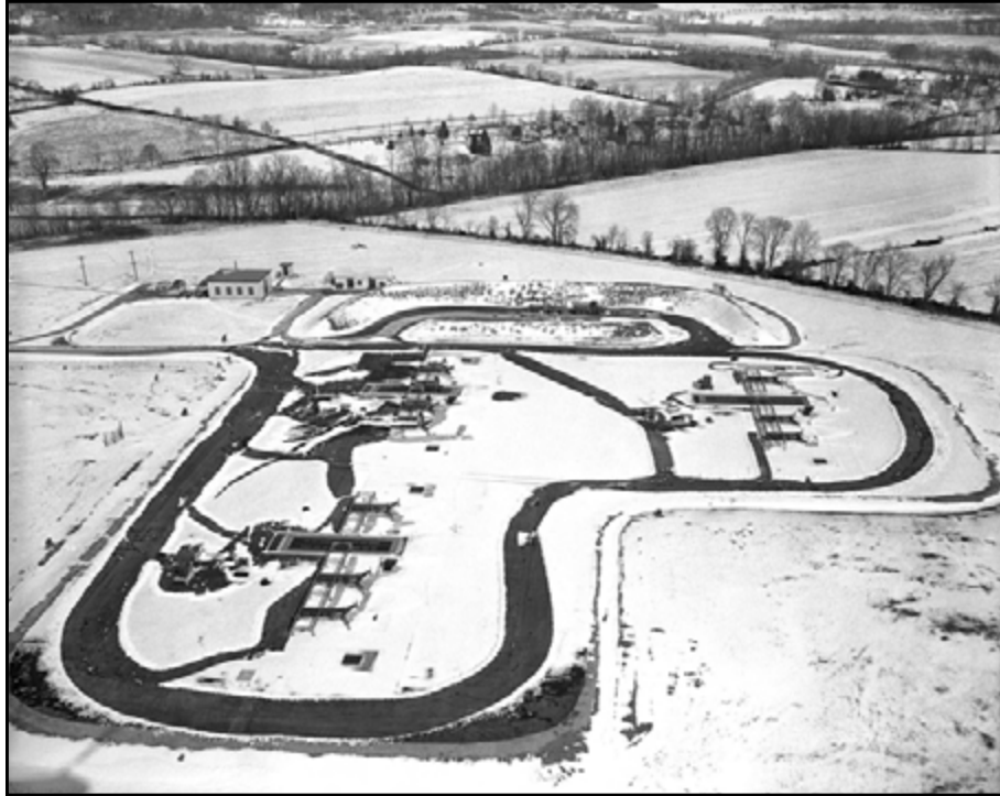
Above: The launch area of PH-82 looking northeast in February 1960. Four Nike-Ajax missiles lie upon their launchers adjacent to the upper left underground missile magazine. The fueling area, with its protective berm, can be seen behind. Courtesy of the National Archives and Records Administration.
